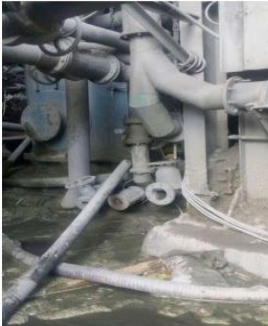
Figure 2: Clean banded area after process modification with auto flush (ZIMEC (2023))
