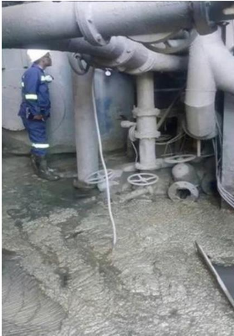
Figure 1: The photo displays a flooded banded area at near a flotation column before modification (ZIMEC (2023))
